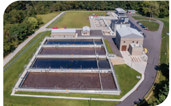
The 4-tank ICEAS SBR system was an ideal solution for meeting nutrient removal requirements and future plant expansion needs
